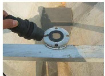
**04. Place the transducer in flange hole**
