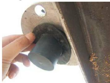
**07. Tighten nuts to fix the transducer**
